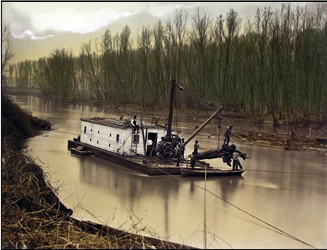
Figure 1. Shows a snag boat removing woody debris on the Great Raft. Photo Credit: Photographic Views of Red River Raft, 1873.
